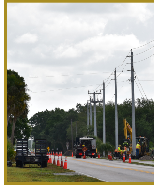
Water Main and Wastewater force main construction taking place along Citrus Blvd. (Photos Courtesy of the Village of Indiantown Staff)
