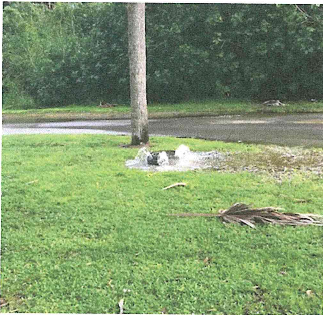
Manhole overflowing raw sewage after heavy rains (overflowed for more than a day)
